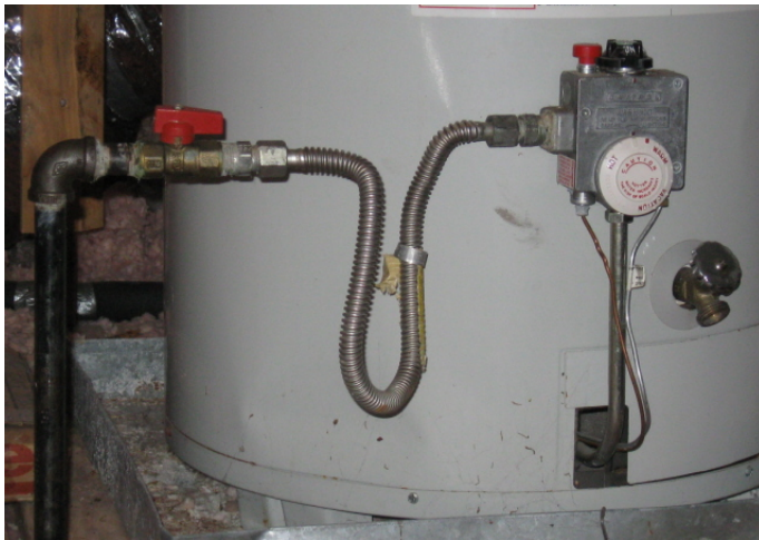
Figure G2419.4(1) SEDIMENT TRAP
