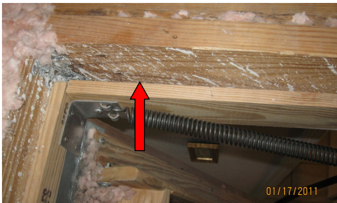
Figure N1102.1.10 TYPICAL SOURCES OF AIR LEAKAGE IN THE HOME
